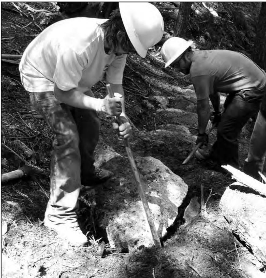
This mountain is the centerpiece of the 36,000 acre Bigelow Preserve. This project is located part-way up the south side of Bigelow. Hand tools such as mattocks, shovels, and pry bars will be used to build waterbars that will divert water from the trail.
