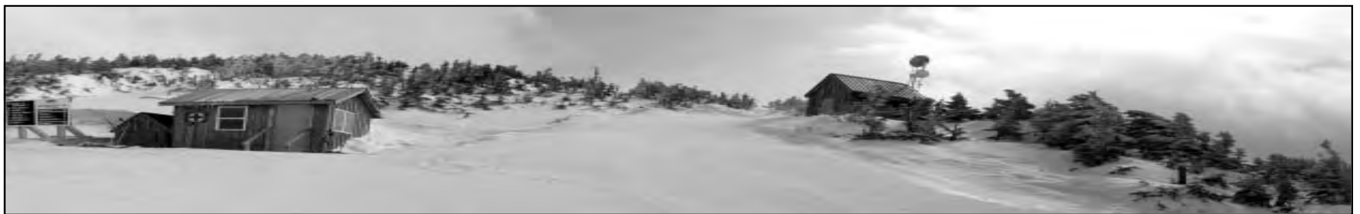
SaddlebackMaine Ski Area replaced the old T-bar to the top of the mountain with a new Quad-Chair lift which operated this past season. The structure housing the lift mechanism as well as the Ski Patrol warming hut are positioned below the ridgeline on the north slope. However, a small communications building with a microwave antenna was constructed higher up the slope. This panoramic photo shows the relative position of this small building in the righthand side of this photo looking up from the north side of the ridge. It is unclear how noticeable (if at all) the structure and antenna are when observed from the AT. Photo and note by Tony Barrett.
