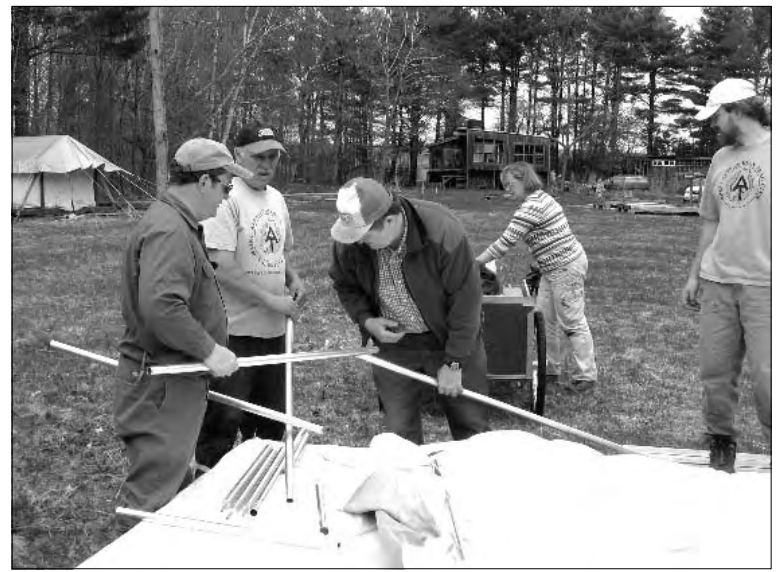
On May 2, a crew of 8 people set up tents at the Garland trail crew Basecamp. A record number of trail crew members are expected to start arriving in Garland next week. Above , Lester Kenway, Ed Langlais, Bruce Grant, Sherri Langlais & Geoff Shadman erecting a tent. Below , Geoff Shadman, Ed Langlais & Lester Kenway are unfolding a tent. Photos by Tony Barrett.
